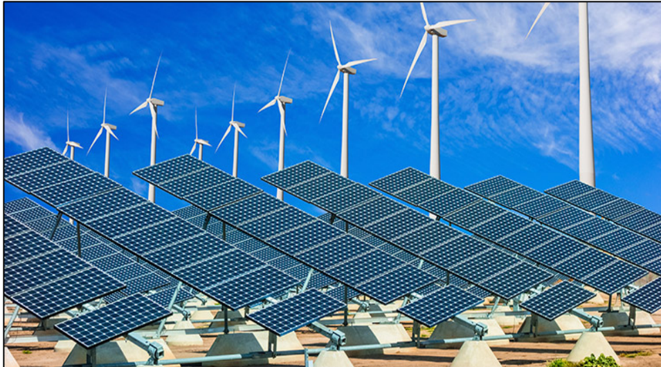
Fig 2. An Image of Installation
