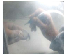
Fig no 4: Sandblasting the coping
