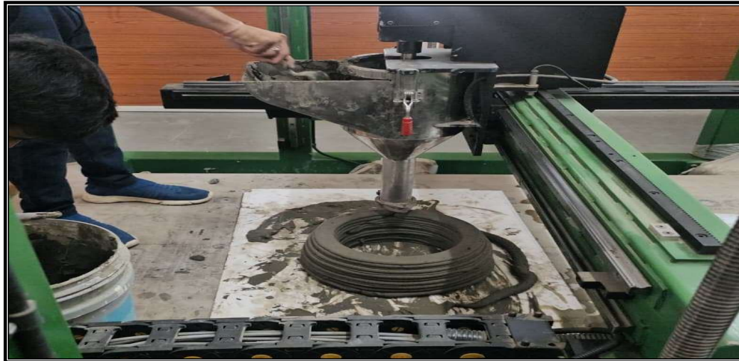
Fig 7: Extruding Process through 3DPC Gantry
