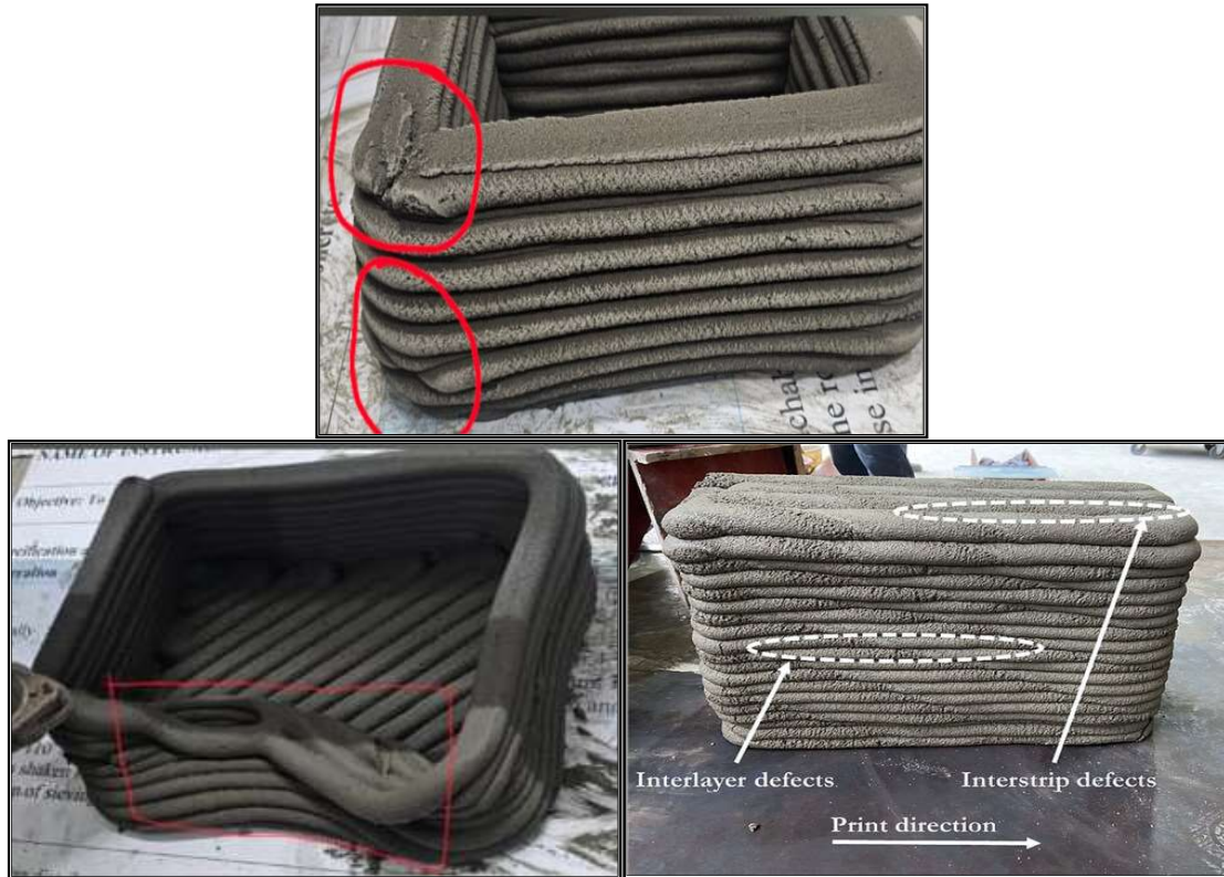
Fig 7: Defects in 3DPC
